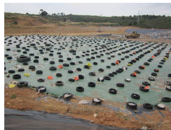
Vista general zona exhaurida
