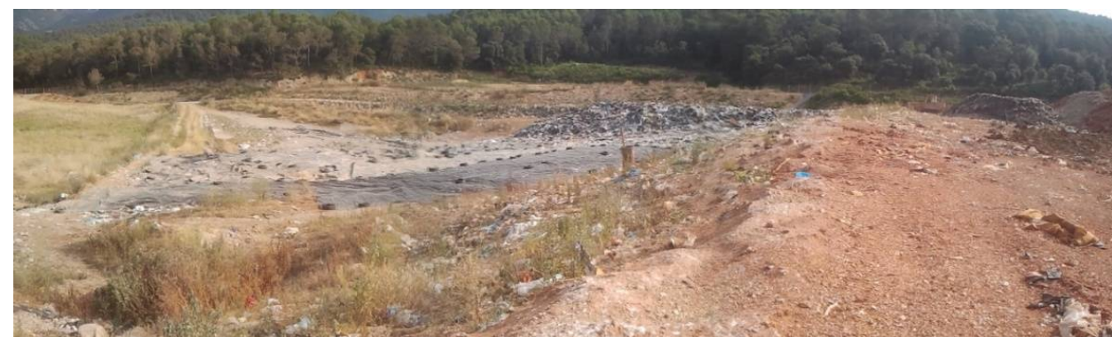
Vista general zona exhaurida
